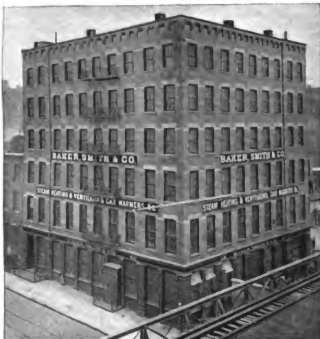
BAKER, SMITH & CO., SOUTH FIFTH AVENUE AND HOUSTON STREET.
